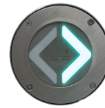
ESCAPE ROUTE TO THE RIGHT
