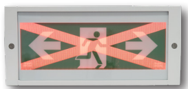
ESCAPE ROUTE BLOCKED
